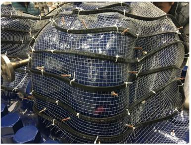
Temperature maintenance of fluid storage vessels with SANTO XPI tracing cable.
